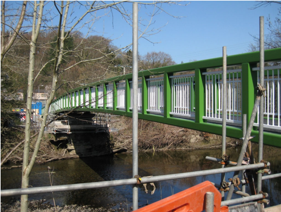
Vierendeel Truss bridge. Green members provide structural strength as well as forming parapet.
