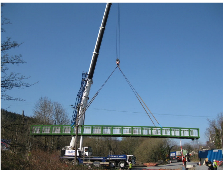
Similar crane size lifting 27m span bridge into place.
