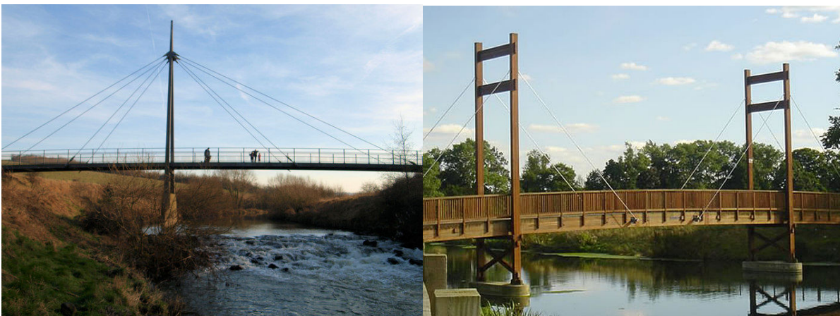
Various styles of ‘Feature Bridge’, Generally dependent on balancing two spans around a support with a cable tower.
