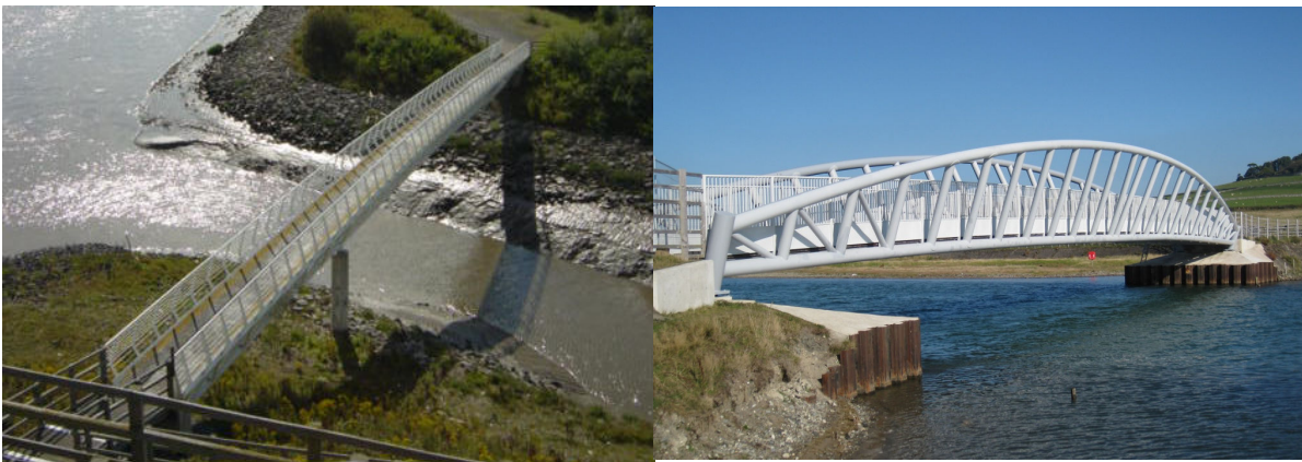
Longer Span ‘Feature Bridges’ using a Light weight triangular truss (Left) or Bowstring Arch Truss(Right).
