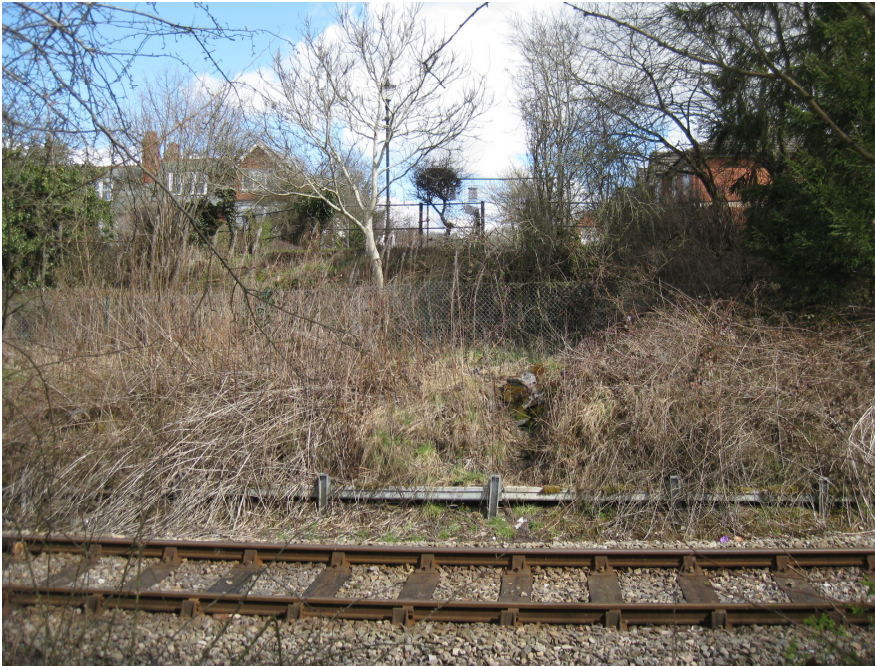
Location of Bridge crossing showing vegetation adjacent to support location
